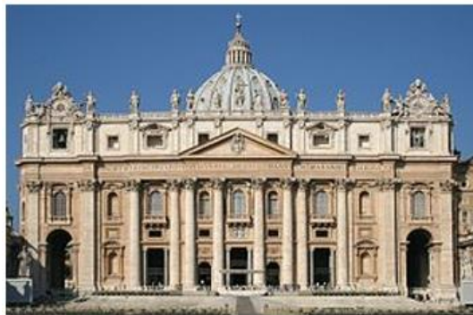
Highlighting the structural elements of the columns outside.
