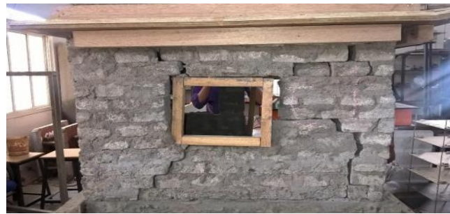
Figure 9: Diagonal cracks developed near window at Shake-9 in model-C1
