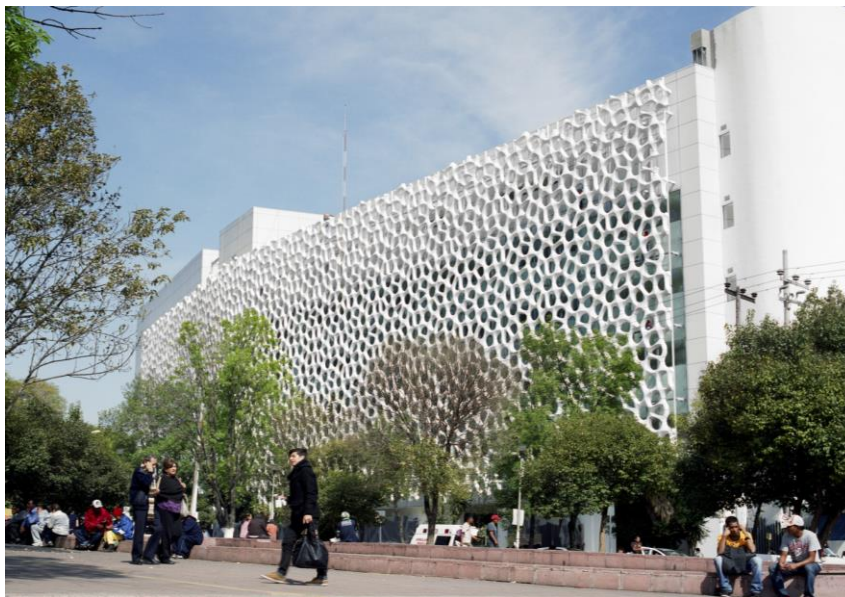
Figure 1. Shows the exterior facade of the hospital 23
