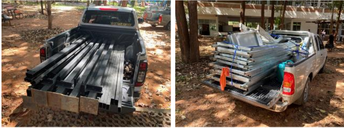
Fig. 5. The elements of the building can be transported by regular small trucks
