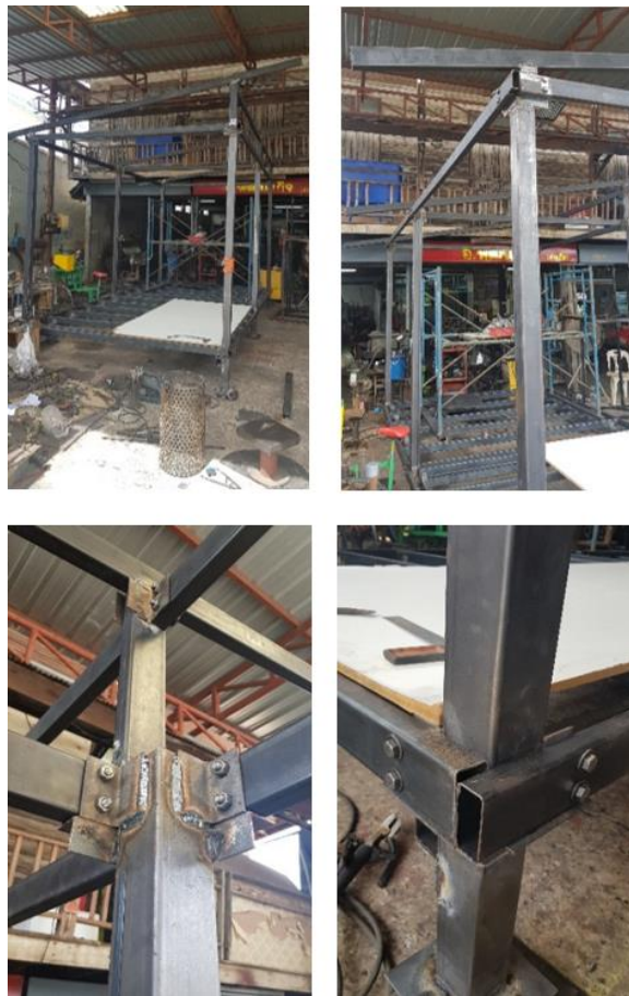
Fig. 6. Installation test at the steel shop
