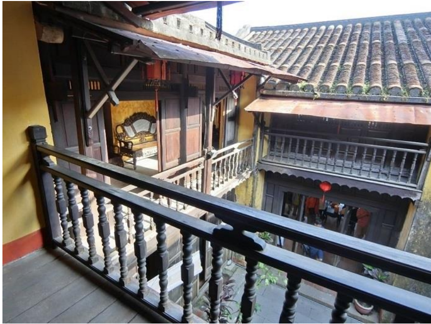
Figure 3. A corner of Tan Ky ancient house, the living room tile roof is roofed in a harmonious yin-yang style, helping to expand the living room space—source: Author Nguyen Thi Bich Van
